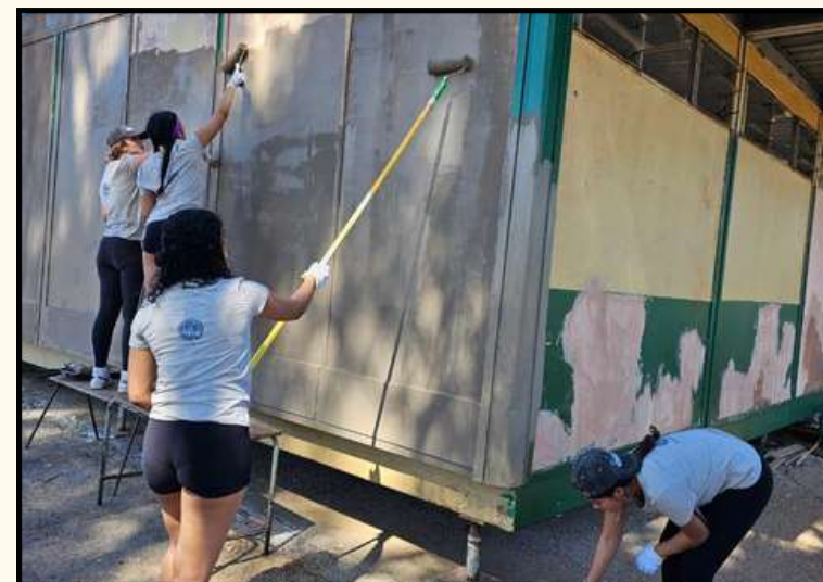
Repainting the outside of the classroom.
