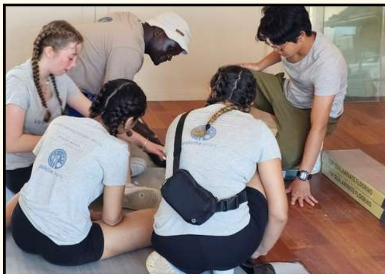
Installment of new wooden floorboards.
